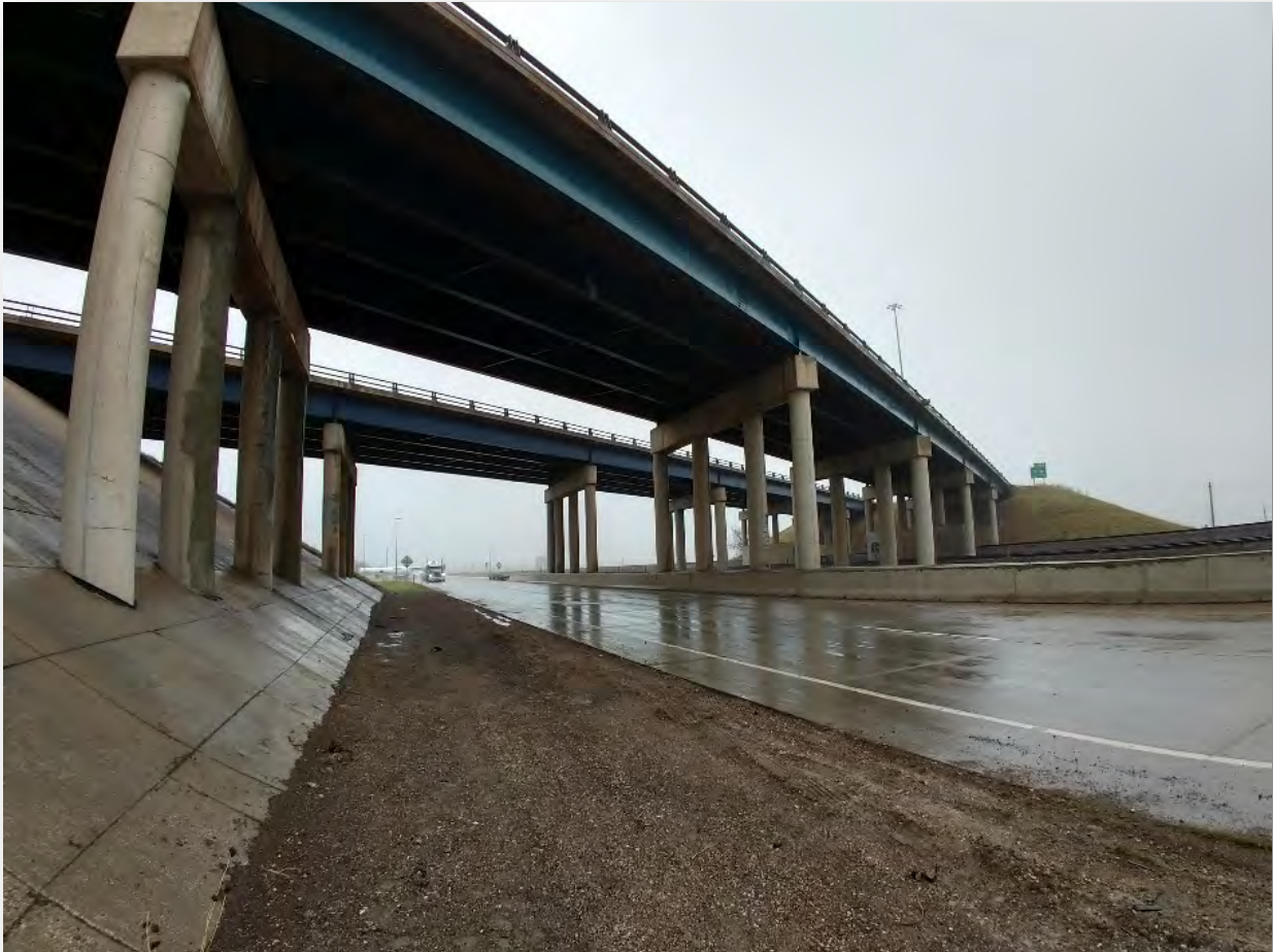
Figure 10 – Existing I-25 Bridges over UPRR
