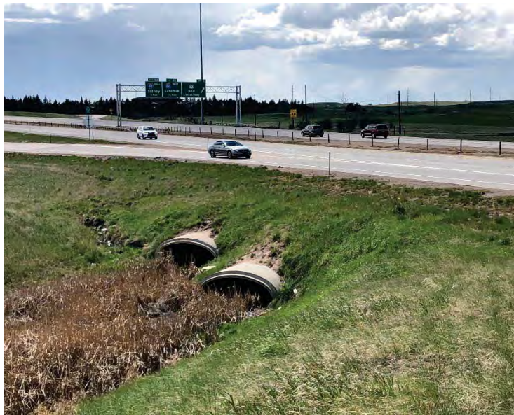
Unnamed tributary to Crow Creek, culverts under I-25 (MP 9.6), looking southwest
