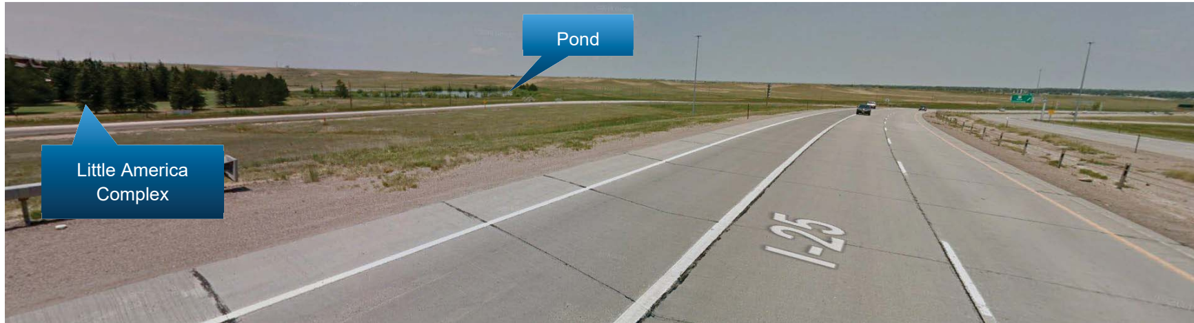
Figure 3-21: View from I-25 Looking North toward Proposed Lincolnway Interchange Replacement
