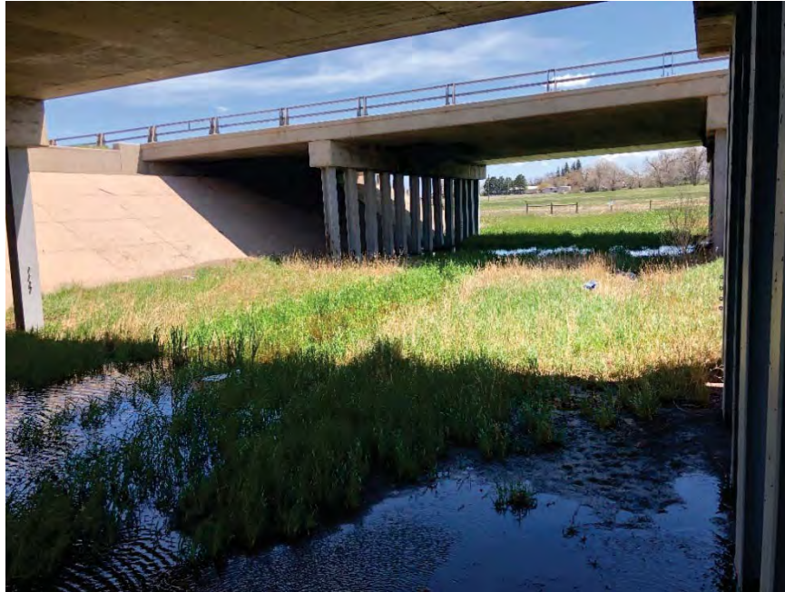
Clear Creek under I-25 bridge (MP 8.4), looking east
